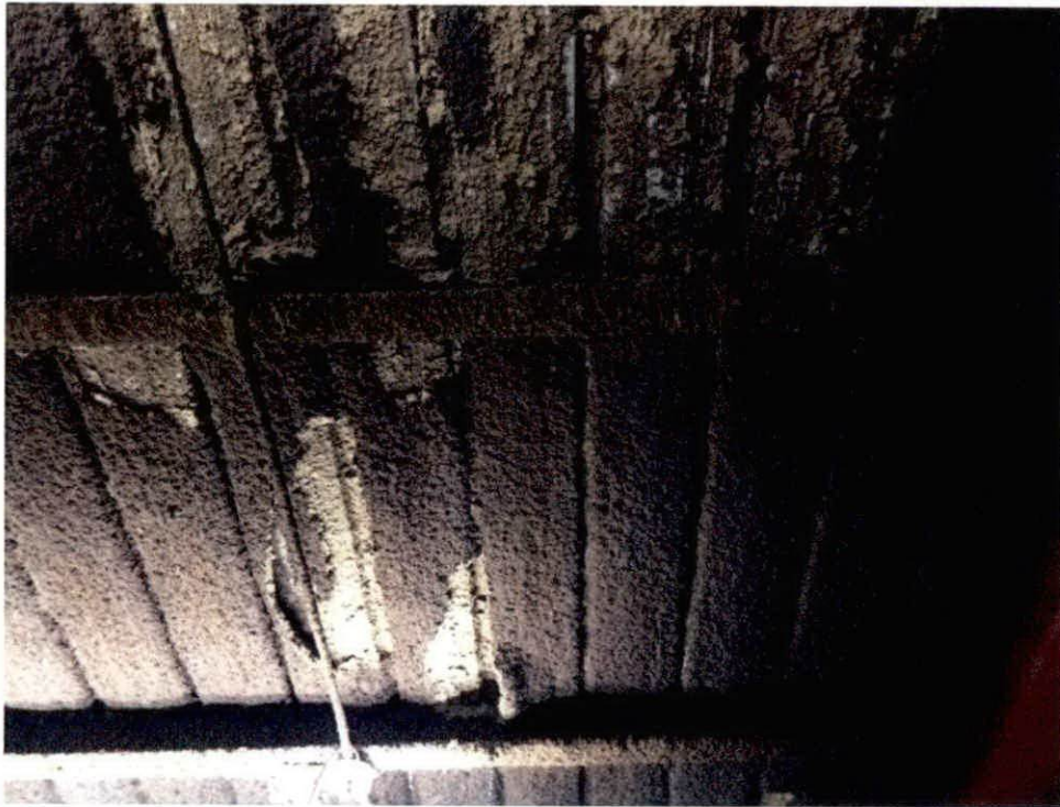
Photo 2: Spray Applied Ceiling Insulation
