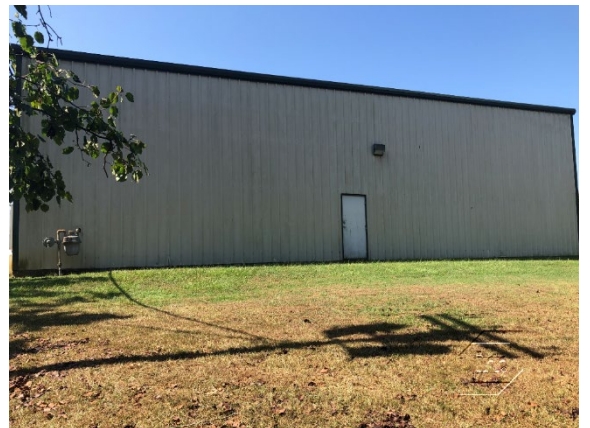
View of North Exterior of Subject (Photo Taken on September 17, 2019)
