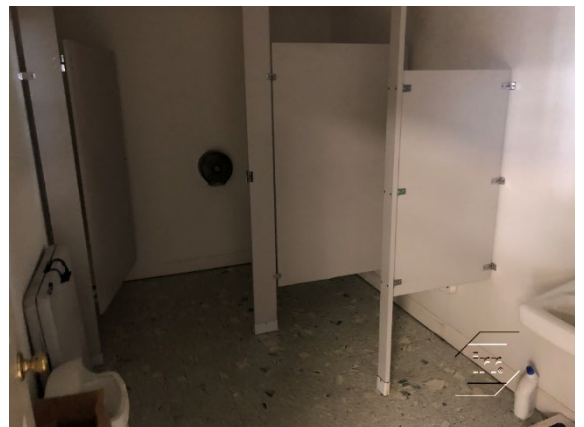
View of Public Bathroom (Photo Taken on September 17, 2019)
