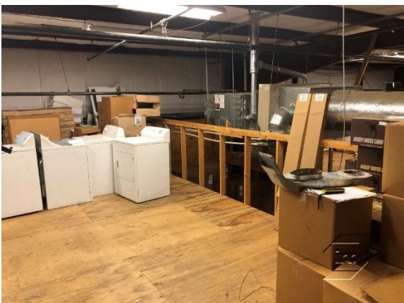
View of Second Floor Storage (Photo Taken on September 17, 2019)
