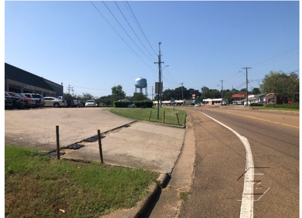
View of Hwy 43 (South) (Photo Taken on September 17, 2019)
