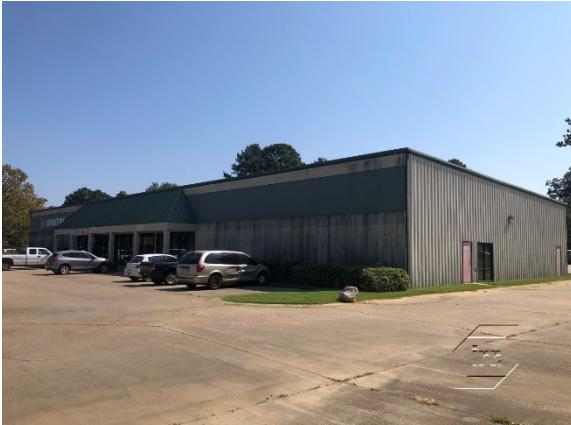
View of SW Corner of Exterior and Parking Lot (Photo Taken on September 17, 2019)
