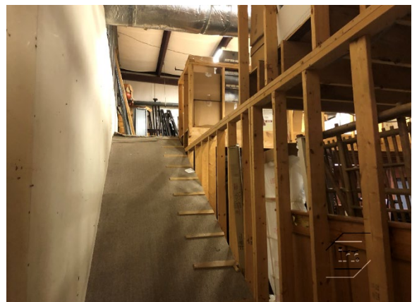
View of Entry to Second Floor Storage (Photo Taken on September 17, 2019)
