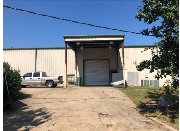
View of Bay Door at Rear of Subject (Photo Taken on September 17, 2019)
