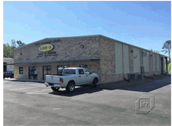
Lease 4 Line - X / Jefcoat Retail/Warehouse Building
