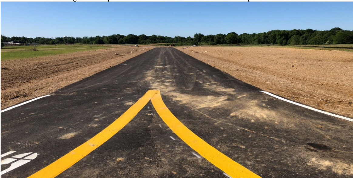
Looking south on Gluckstadt Way from Church Road
