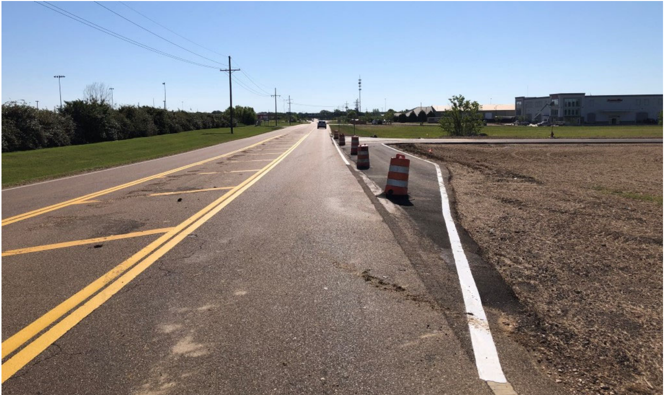
Looking east on Church Road at new Gluckstadt Way intersection.
