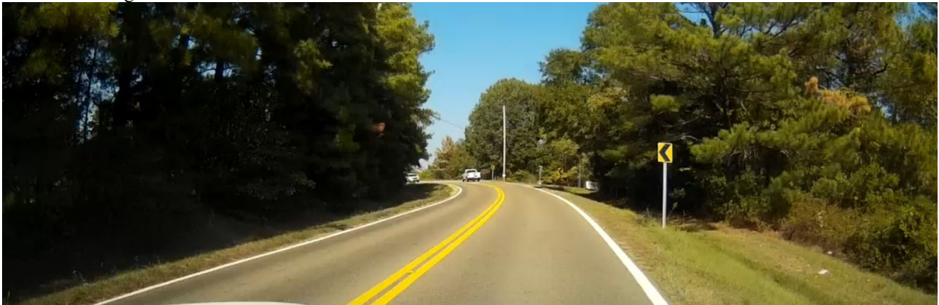
Below: Looking north on Catlett Road at horizontal curve.
