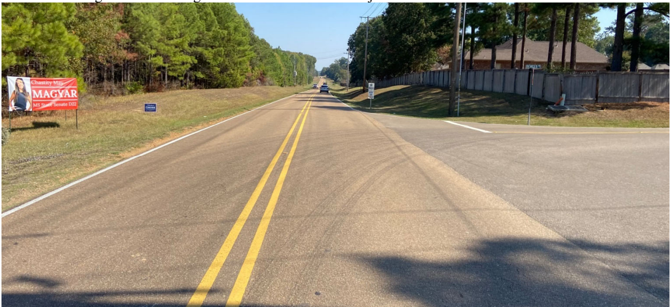
Below: Stribling Road – Looking east across Dewees Road adjacent to Fire Station.
