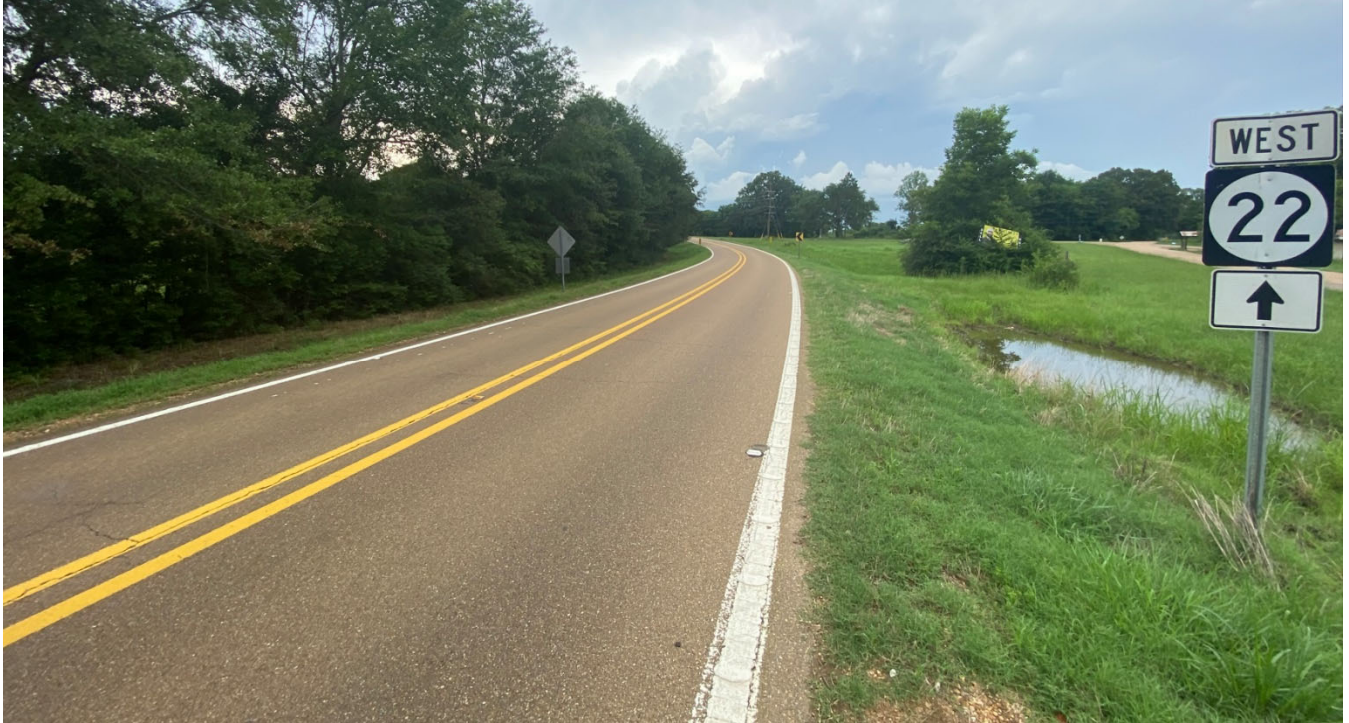
Above: Looking north on Livingston Vernon Rd at MS Hwy 22 intersection. Stop line at 45 degree angle to traffic. Below: Looking west on MS Hwy 22, just west of Livingston Vernon Road. Southern tree line limits sight distance.
