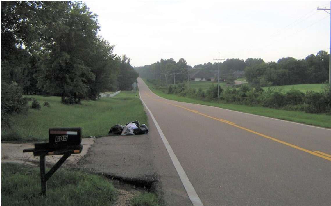
Above: Looking north on MS Highway 463 from north of the vertical curve on Gluckstadt Road.
